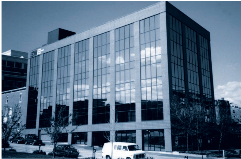
Bottom: Office building at 261 Commercial Street, Portland, Maine, where MEMIC moved its headquarters in September 1993.
